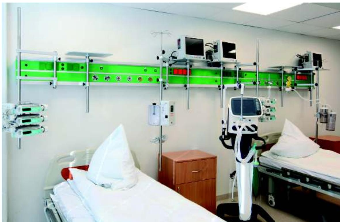
Wall pendants can be joined end-to-end to form a continuous module for general resuscitation rooms and intensive therapy wards
