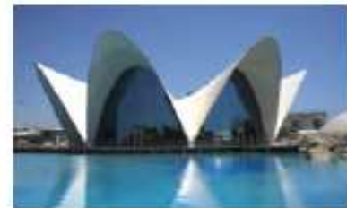
Oceanographic Park, Valence – Spain Santiago Calatrava Architect
