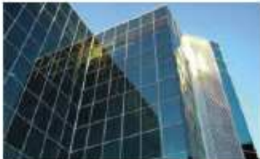
Cristalia Business Park, Madrid – Spain Rafael De La Hoz Architect
