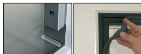
Rounded internal corners
